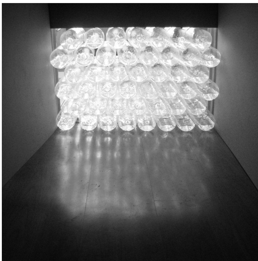
Figure 1. The diffuse light passing through a simple stacked wall made from reused PET bottles due to the multiple reflections generated by the honeycomb structure
