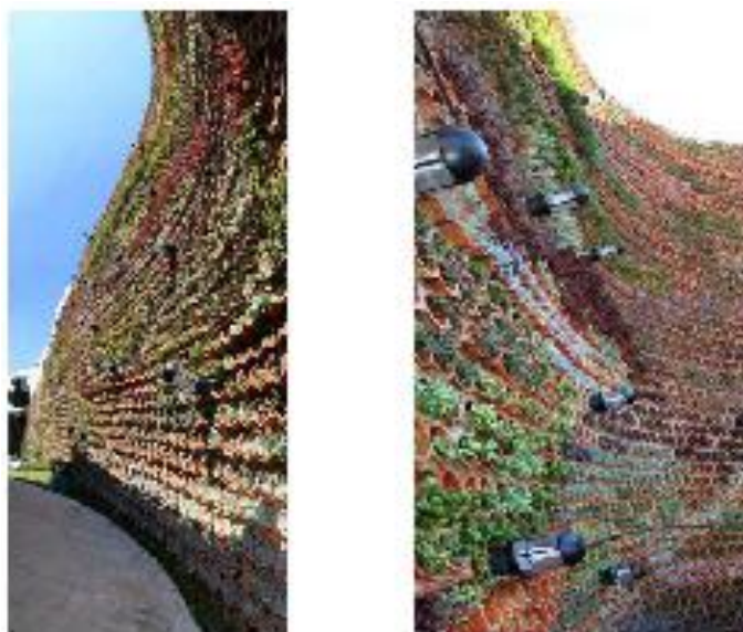
Figure 12. An example of the fence acting as a noise barrier
